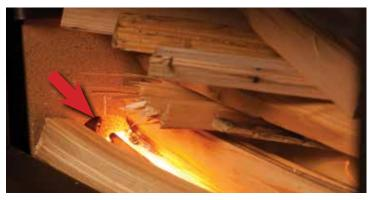
2 A compressor will force 1,400 degree preheated air into the firebox directly onto the wood, giving a clean, fast, smoke-free start up within 30 seconds.
